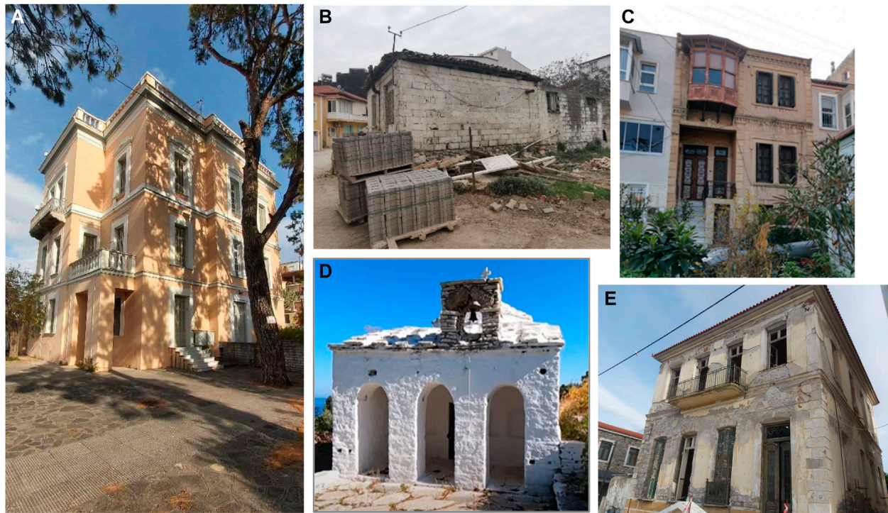
FIGURE 13 | Examples of masonry building stock in the affected areas [(A,D,E) in Samos, (B,C) in Izmir].
