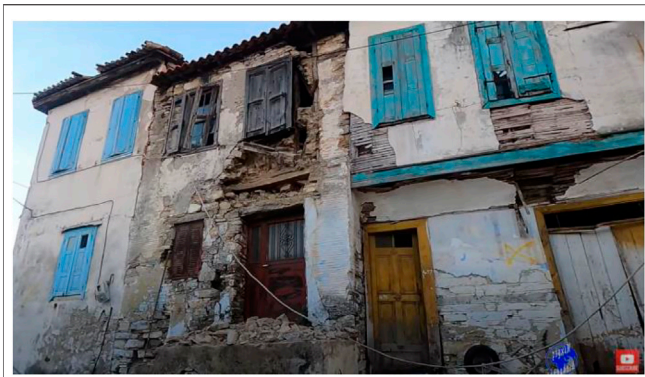
FIGURE 15 | Examples of stone infilled (building in the middle) and bağdadi clad (building on the right) timber-masonry homes (in Samos, picture from Mikres Diadromes Samou, 2020).
