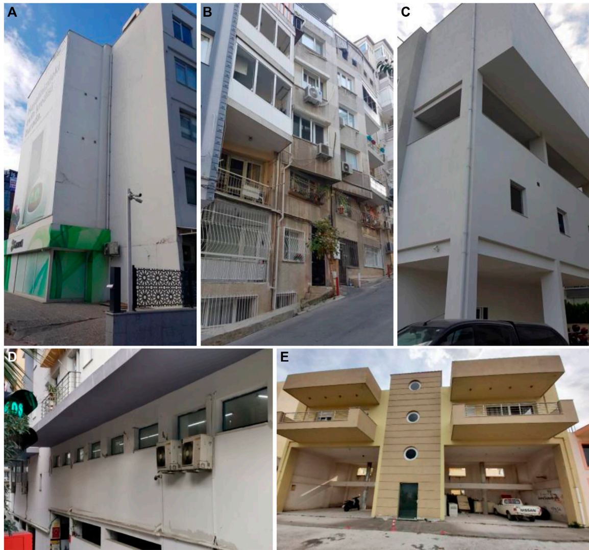
FIGURE 12 | Examples of common irregularities in RC buildings [(A): Changes in stiffness due to structures attached to the main building, (B,C): Elevation and plan irregularities, (D): short columns, (E): plan and elevation irregularity, and large openings at the ground floor].
