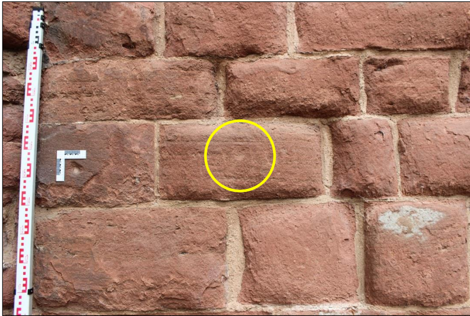
Figure 4: Photograph of a possible impact scar remnant at Chester, Cheshire. The remnant is located in the centre of the circled area
