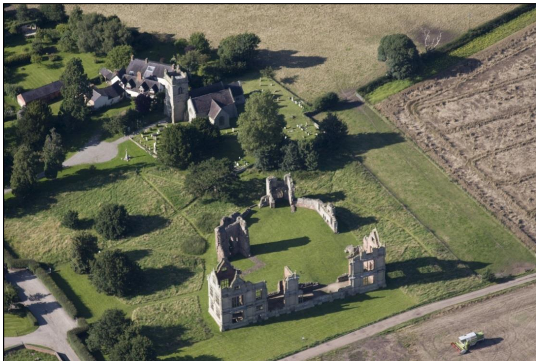
Figure 63: Photograph of Moreton Corbet Castle ruins and adjacent St. Bartholomew's Church. Image taken by Mick Krupa. ©Shropshire Council
