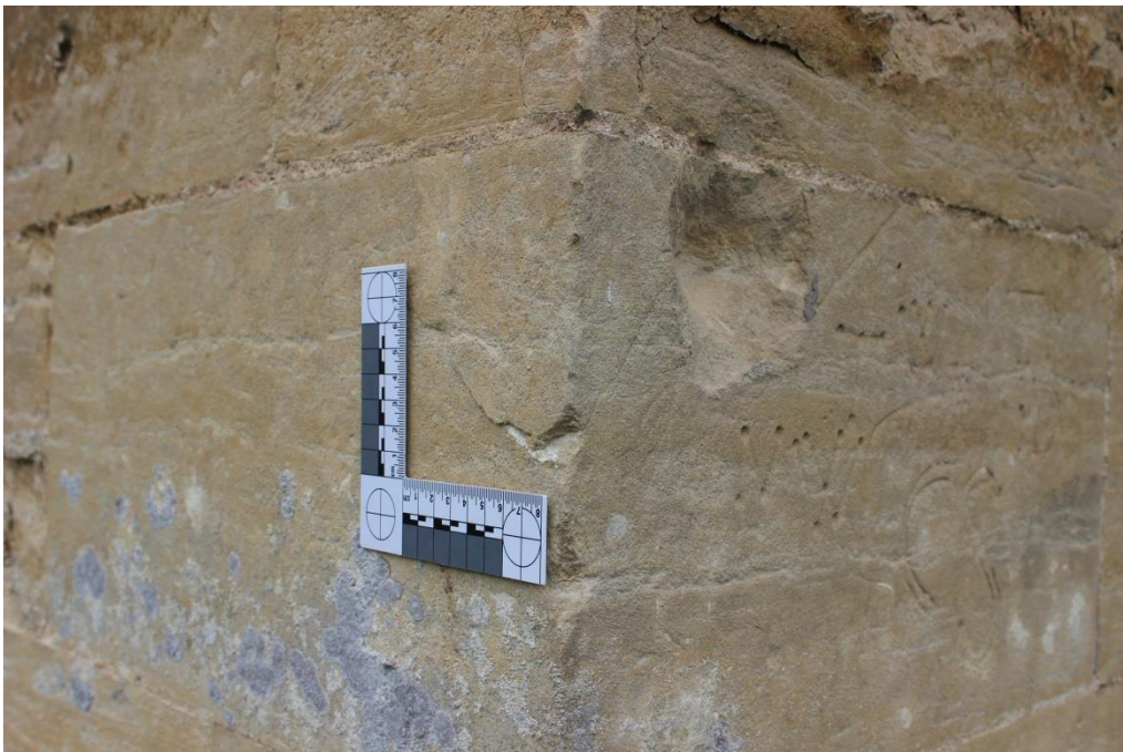
Figure 10: Photograph of an impact scar from Hillesden church, Buckinghamshire, showing a radial fracture emerging from an adjacent surface of the impacted block
