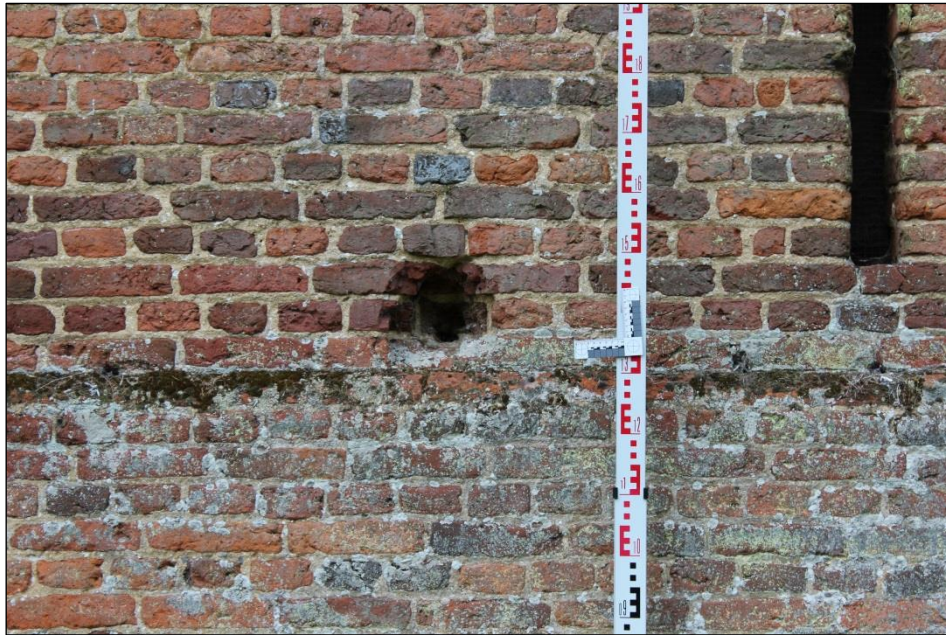
Figure 14: Photograph of artillery impact on brickwork at Basing House, Wiltshire
