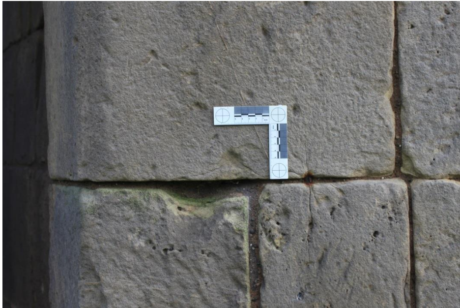
Figure 11: Photography of an impact scar surrounded by numerous features that mimic aspects of early modern small-arms impacts
