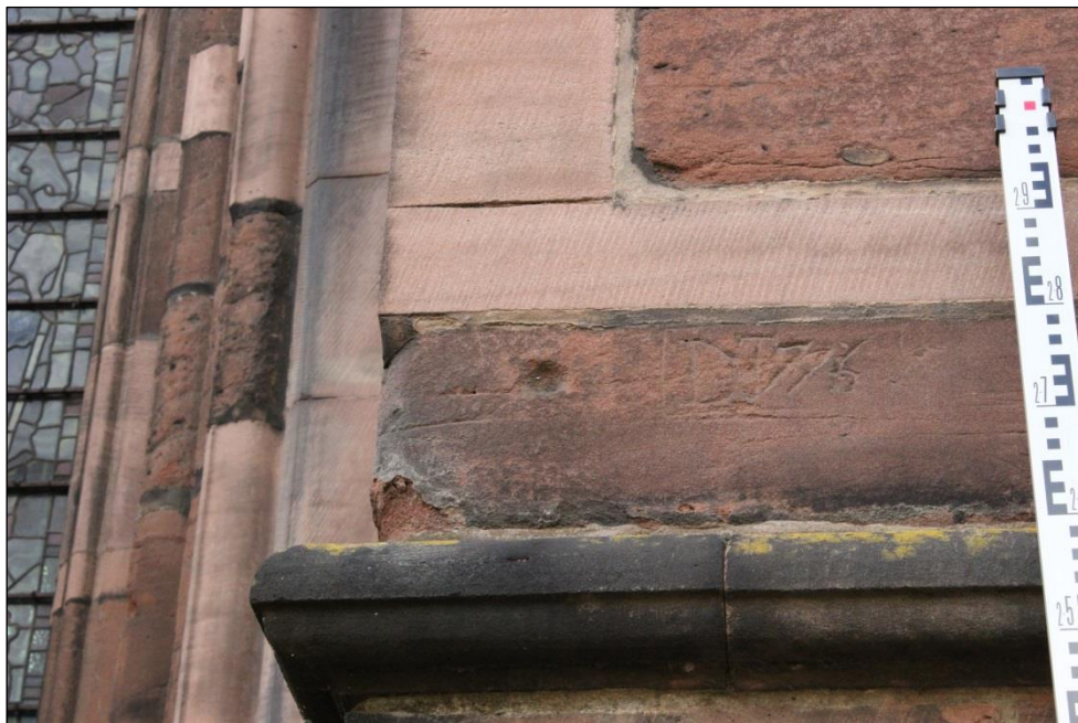
Figure 5: Photograph of stone replacement adjacent to an impact scar at Chester Cathedral
