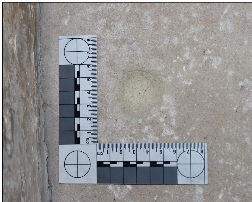
Figure 84: Internal scar in the squire's pew at St. Bartholomew's Church, Moreton Corbet. The scar shows the same internal cup-shape as seen elsewhere, and lighter stone in the base of the scar in comparison to the case-hardened patina on the block surface
