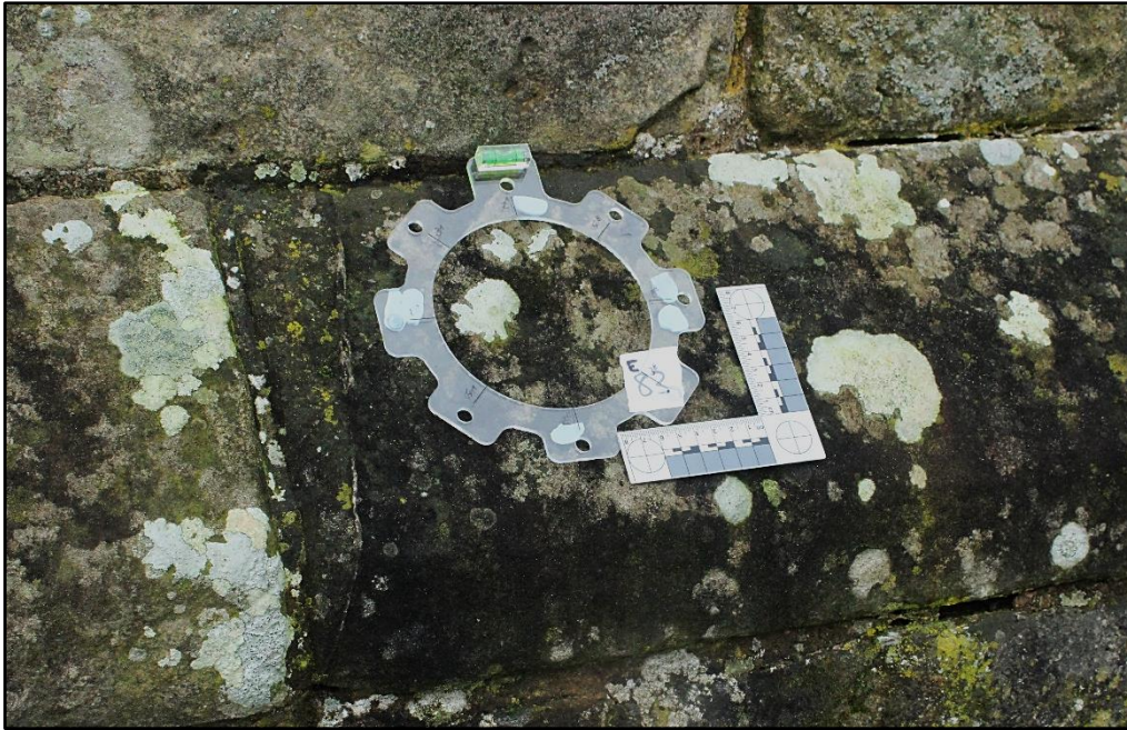
Figure 79: Impact scar E83 located on backwards-sloping wall surface on Moreton Corbet Castle
