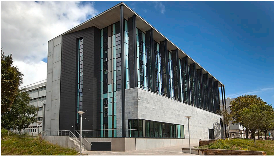
Fig. 1. Marine Building located on the University of Plymouth campus [32].
