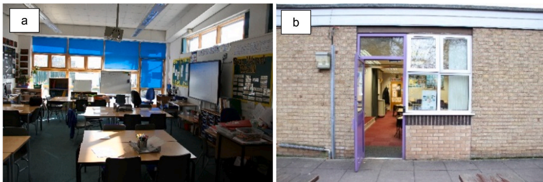
Fig. 2. Windows and external door in school 3, classroom 3.10 (a) and school 4, classroom 4.14 (b).
