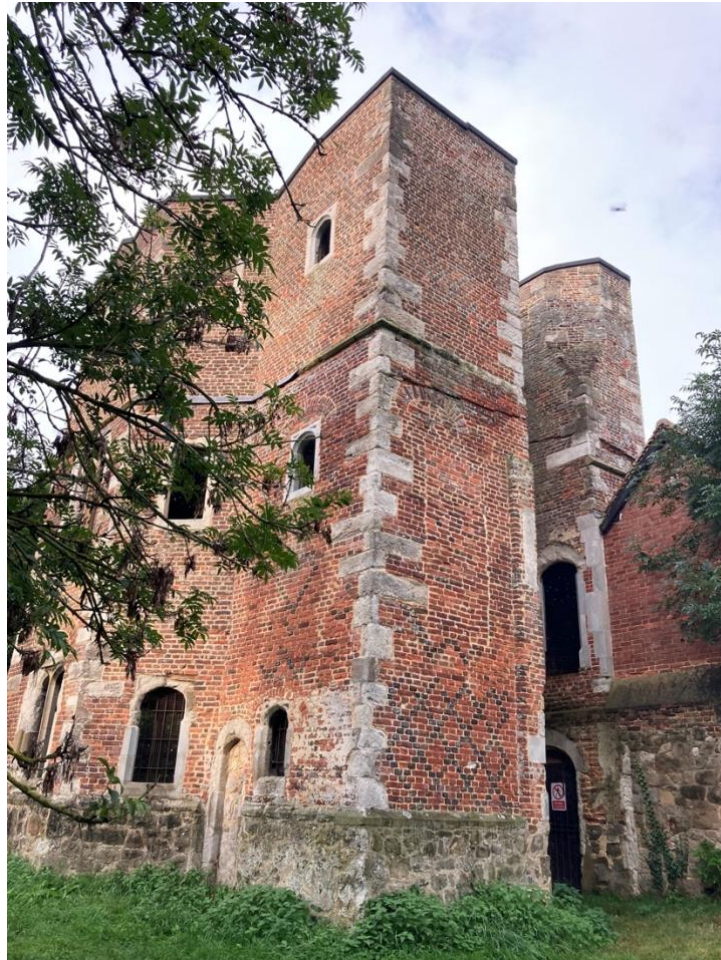
Figure 7. The remaining and unoccupied sections of Otford Archbishop's Palace © Christopher Moore
