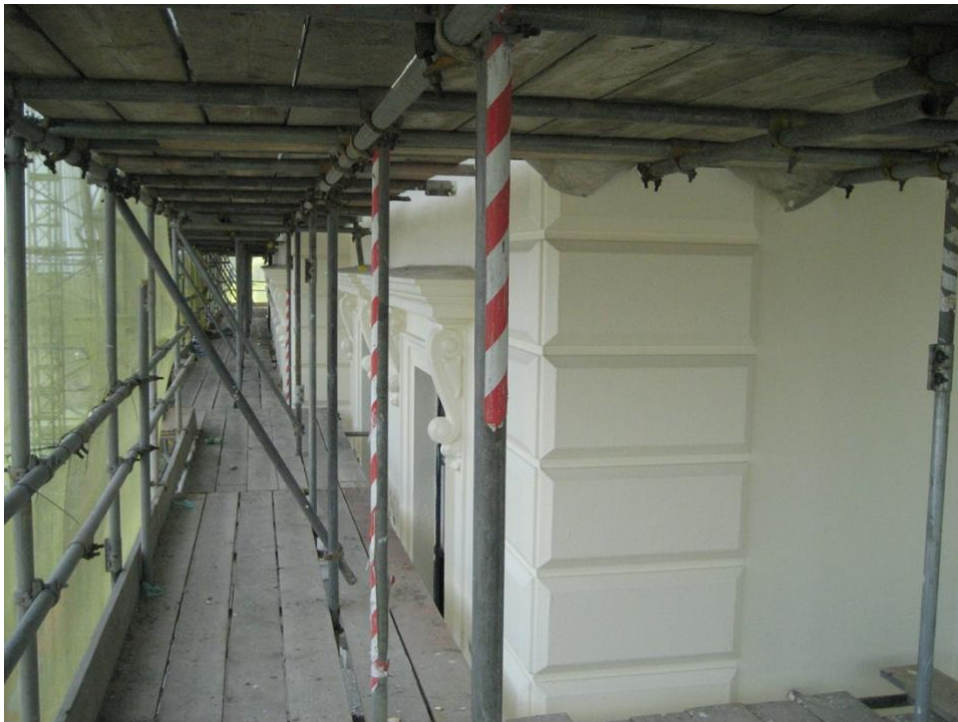
Figure 41. Works to a listed building in Dover, 2020 © Christopher Moore
