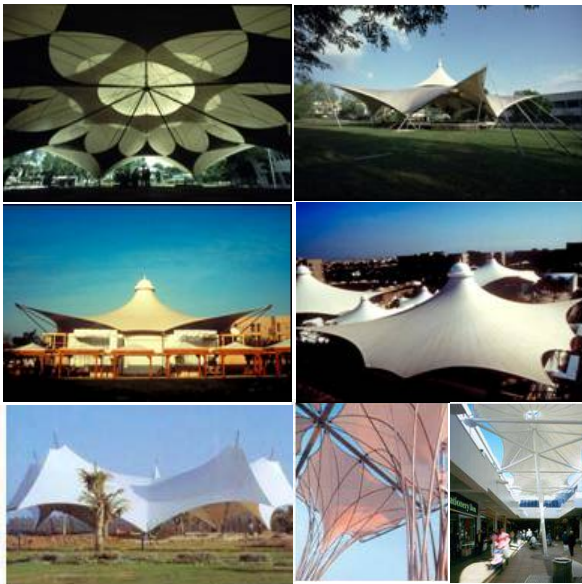
Figure 12 Photos depict different fabric membrane structures for opened, semi-enclosed, and enclosed space as microclimate modifiers
