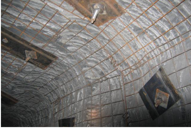
Fig. 3. Surface condition in the mine working with roof bolting
