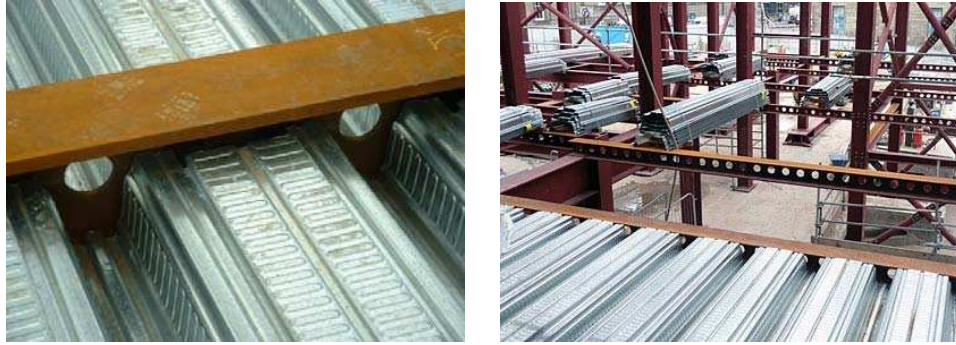
Figure 2. USFB construction adopted by Westok Ltd.
