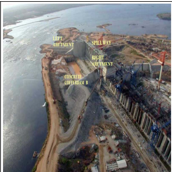
Fig. 2. Aerial Photograph of Caruachi Dam (Abutment details)
