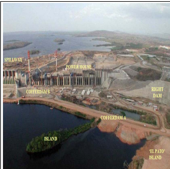
Fig. 1. Aerial Photograph of Caruachi Powerhouse and Civil Works
