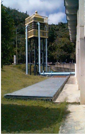
Fig. 1. Underground and Elevated Open Tanks
