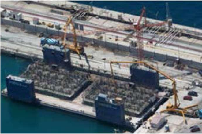
Figure 1. Real construction process.
