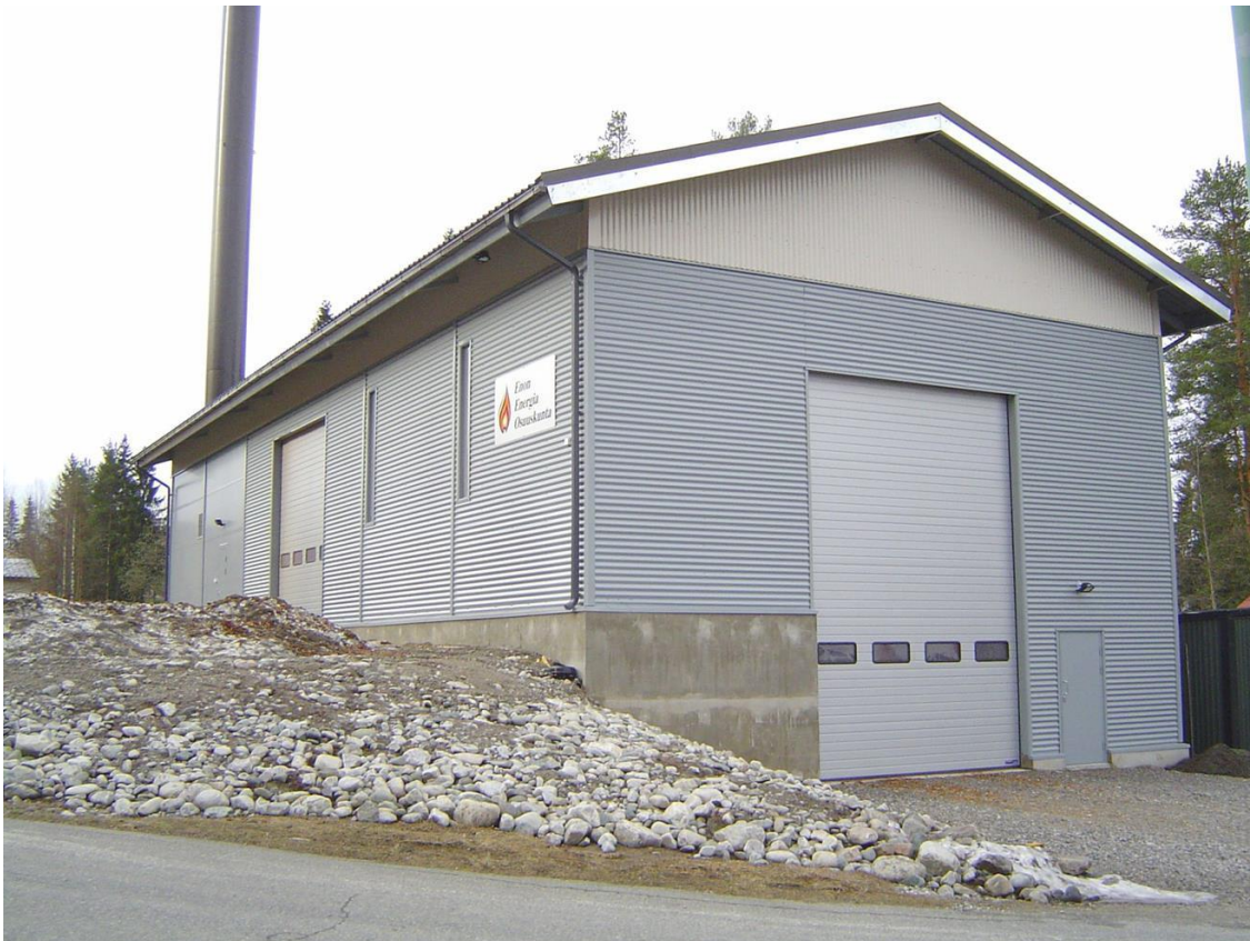
Picture 4: Eno Energy Cooperative, Alakylä heating plant. Photo: Eno Energia.
