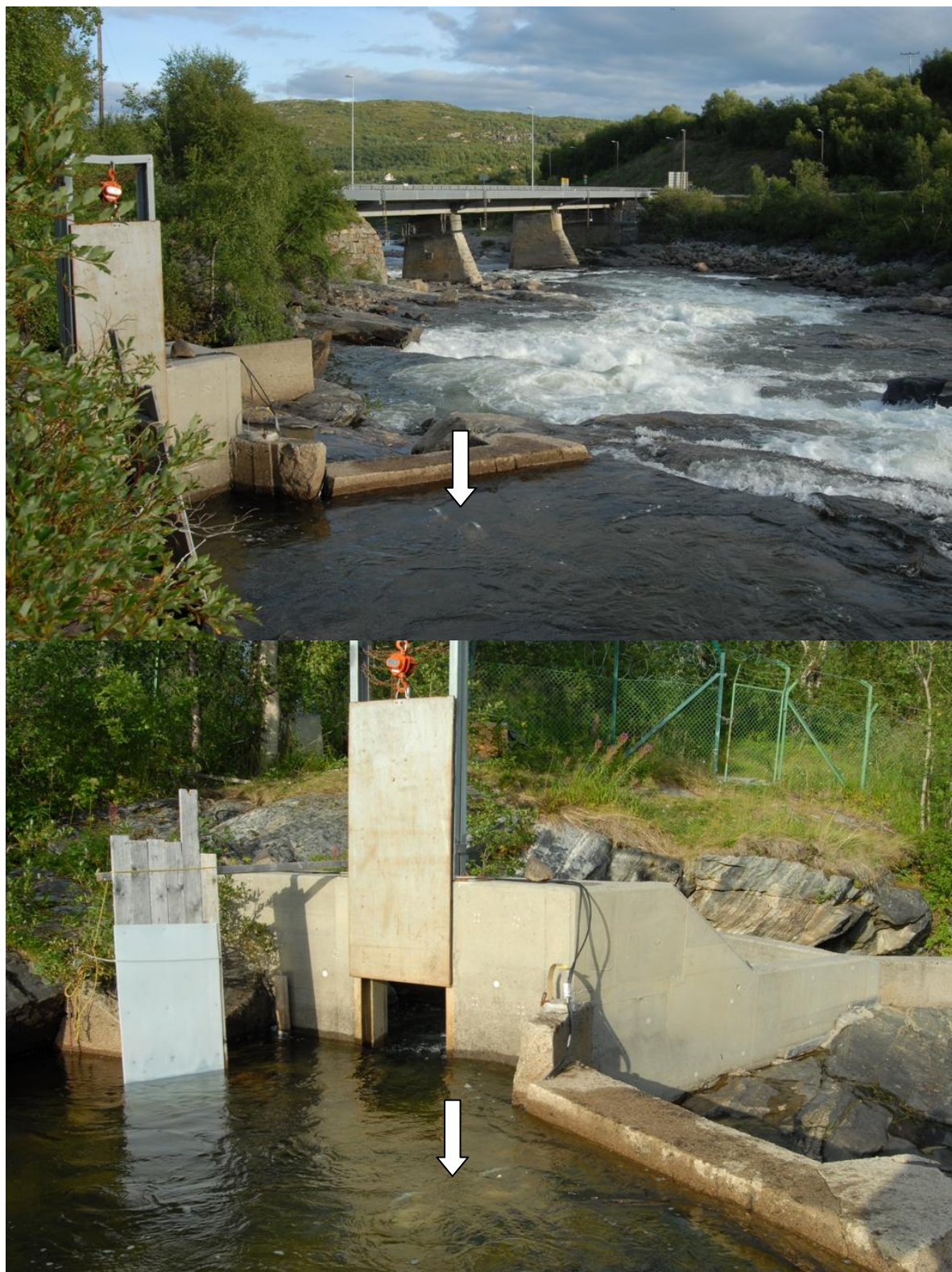
Figure 2. Installation of the underwater camera and halogen light (arrow) above the Skoltefossen fish ladder in the River Neiden. Photos: P. Orell.
