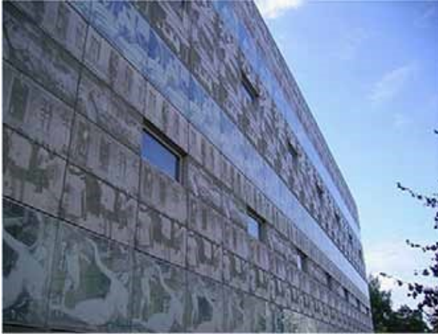
Figure 2. Herzog & De Meuron. Library of University of Applied Sciences in Eberswalde (1999). The image shows the effect of “textilization” of glass and concrete. Photo: Immanuel Giel (August/2005) [CC BY-SA ( http://creativecommons.org/licenses/by-sa/3.0/ )] source: https://commons.wikimedia.org/wiki/File:FH-Eberswalde_Bibliothek_Fassade.jpg (downloaded on 1/4/2020)
