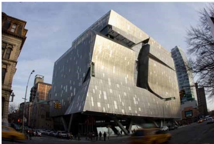
Figure 3. Morphosis Architecture, with Gruzen Samton as associate architect. Cooper Union New Academic Building, Cooper Square, New York City (2009). The image shows the transformation of a cube block. Photo: short.dale [CC0] (April 2011) source: https://commons.wikimedia.org/wiki/File:CooperunionNAB.jpg (downloaded on 1/4/2020)
