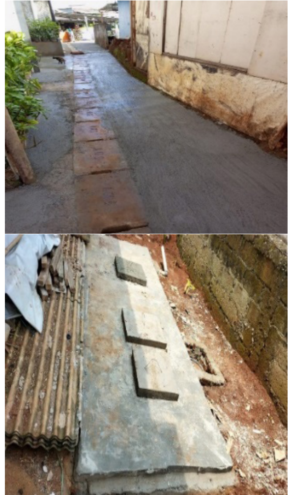
Figure 3. Construction of Sanitation Facilities and Roads in Depok Village in 2018
