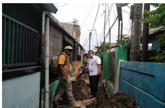
Figure 2. Road Construction in Depok Village in 2021
