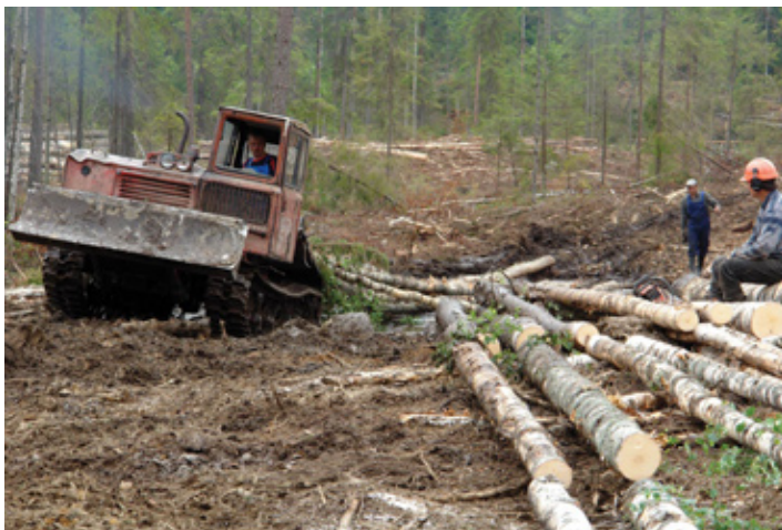
Figure 9.7. Cable skidder. (Vasiliy Katarov)
