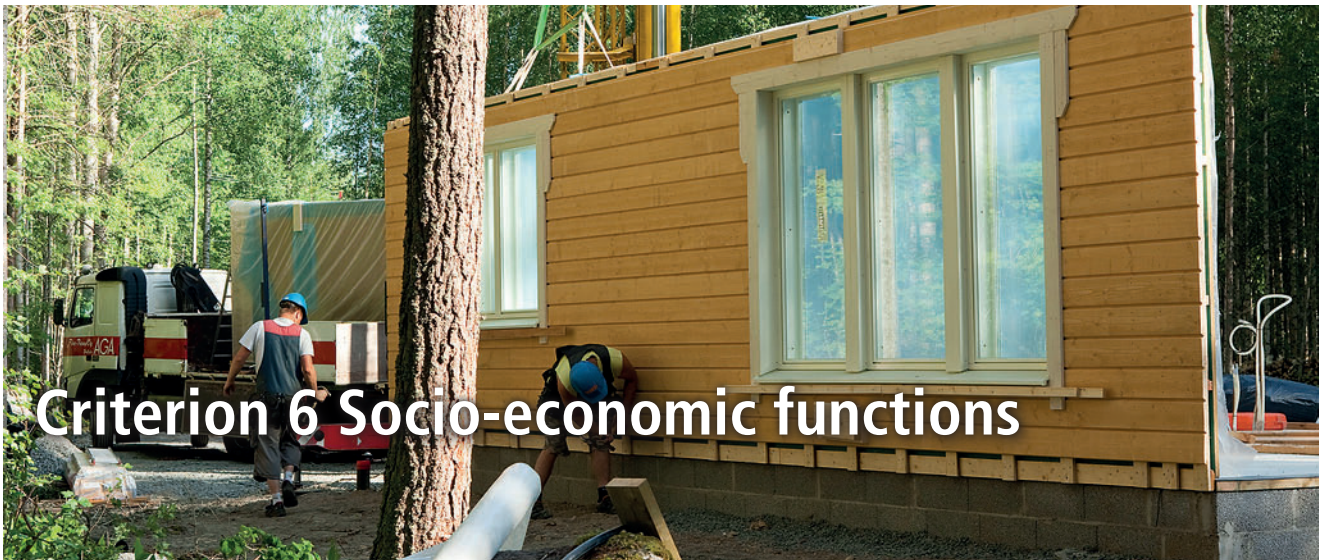
Installation of wooden wall elements for a private single house.
