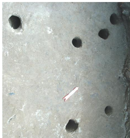
A photographic view of a section of the postholes in layer 9. Author's photo, 2008
