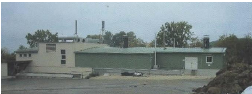
Figure 11.9. BGP 53, left: building for the CHP with gas torch, middle: gas storage, right: digestate separator (FNR 2009).
