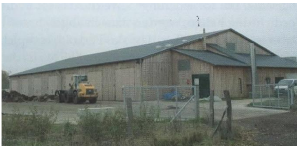
Figure 11.11. BGP 62, building with seven box digesters (Source: FNR 2009).
