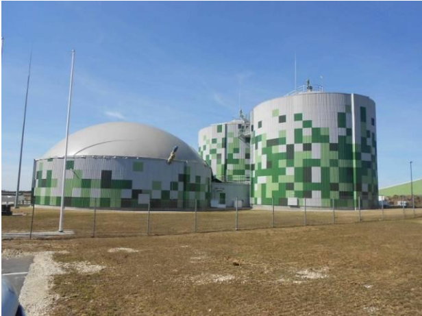
Figure 9.1. Aravete biogas plant (picture by Tauno Trink).
