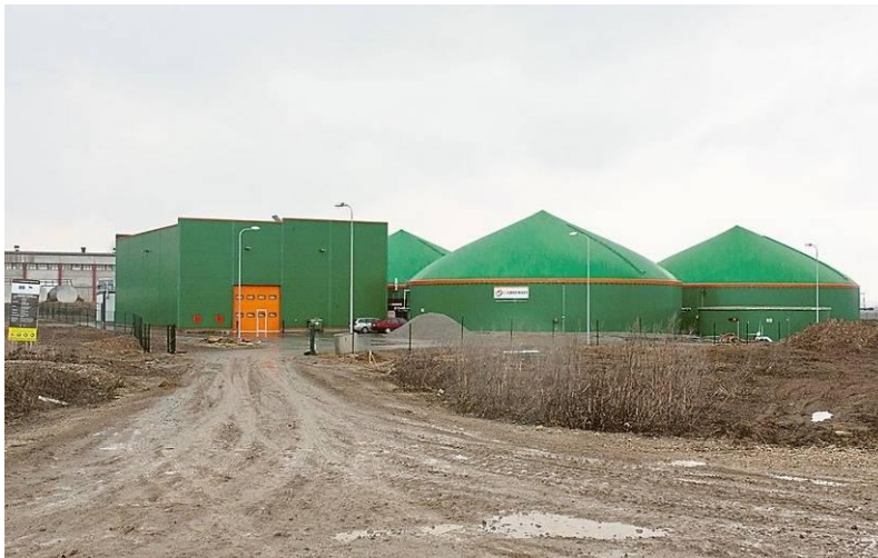
Figure 9.3. Vinni biogas plant (picture by Ain Liiva).
