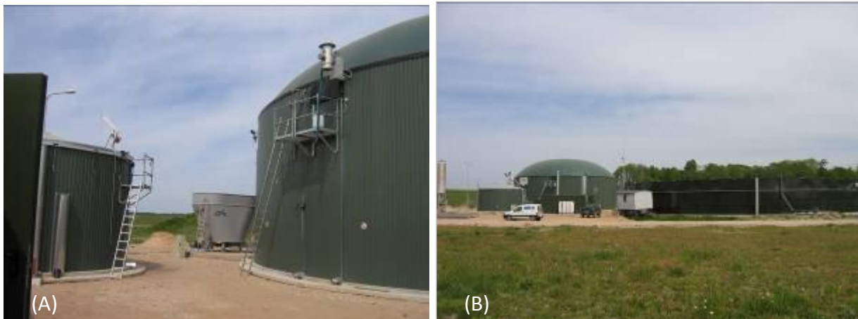
Figure 6.3.3. Biogas plant in dairy farm Līgotnes: (A) Anaerobic digester (2000 m 3 ) on the left; (B) anaerobic digester and digestate storage tank (4000 m 3 ).
