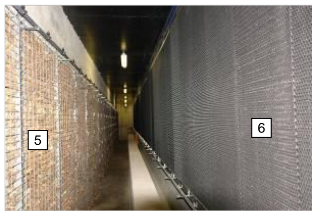
Figure 6.3.10. Air filtration system: 1) water supply pipes with sprinklers; 2) plastic cell wall; 3) ventilators; 4) wall of barn; 5) wood shavings filling; 6) plastic cell wall.
