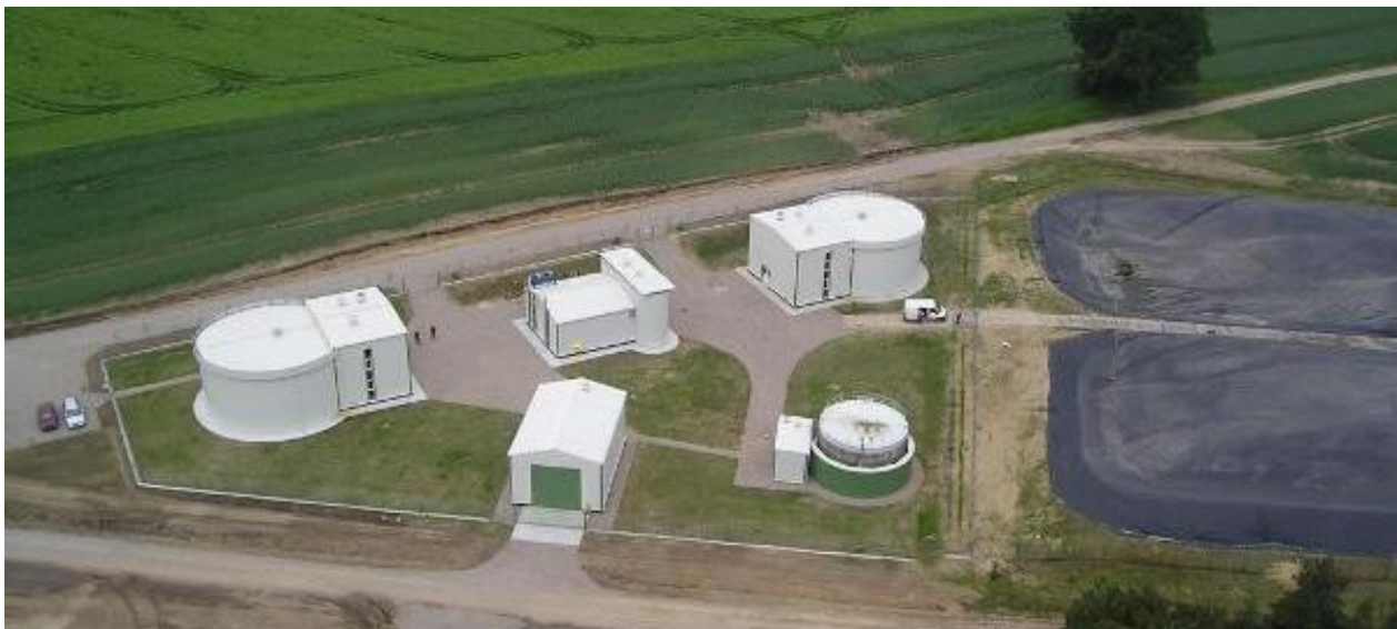
Figure 6.5.13 Biogas plant on Farm 1 (source: POLDANOR).
