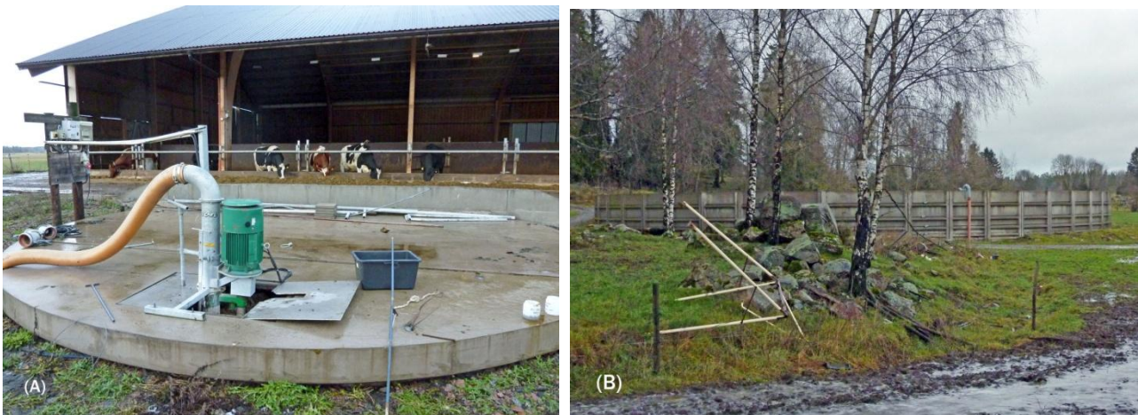
Figure 6.6.3. Pictures of A) temporary storage tank (MP2) that is immediately adjacent to the housing unit (H2), and B) storage structure S1 including filling pipe for slurry pumped from MP1.
