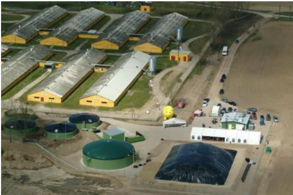
Figure 6.5.17. Biogas plant on Farm 4 (source: POLDANOR).
