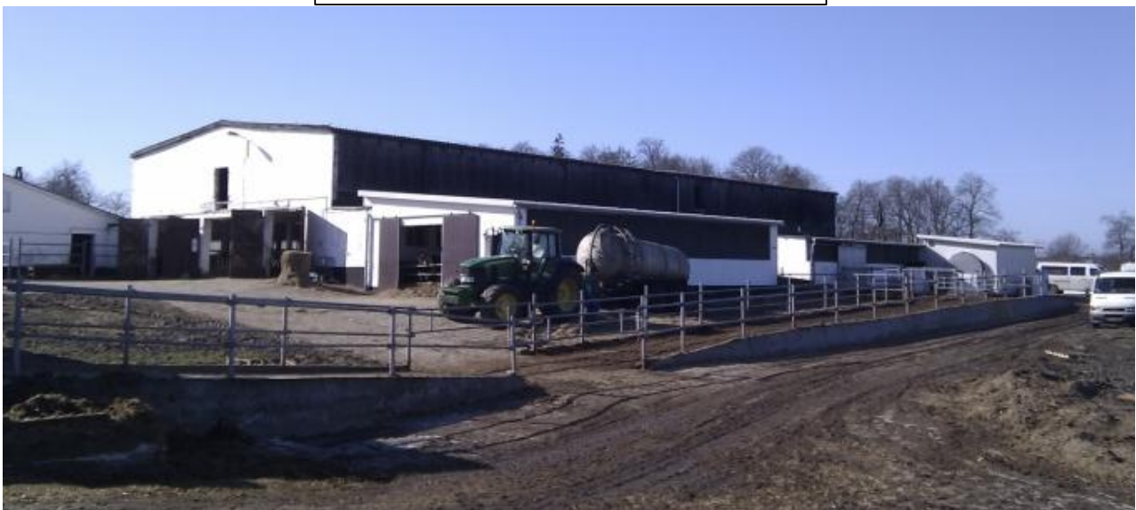
Figure 6.5.7. Barn 1 and 2 with loose housing in open pens (System 1), only one barn shown.
