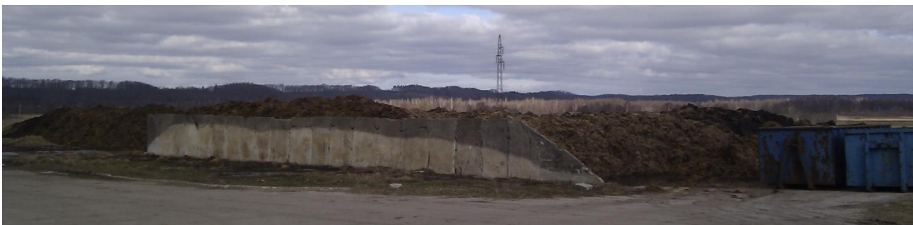
Figure 6.5.4. Outdoor concrete pad for solid manures from System 1 and 2.
