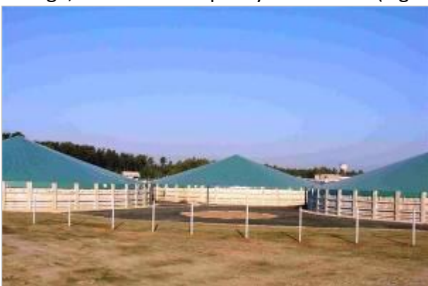
Figure 6.3.11. Covered slurry tanks.
