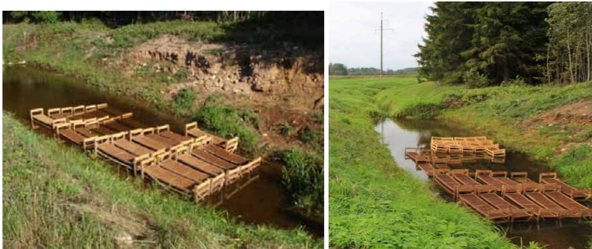
Figure 16. Stacked filter elements at Rahinge site no 1. Photographs by Egle Saaremäe and Indrek Talpsep.
