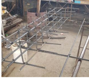
(a) Reinforcing bar assembly
