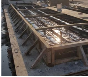
(c) Reinforcement bar and tendon placement (B,U, and G)
