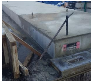
(h) Removing formwork
