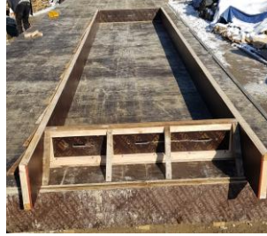
(b) Wooden formwork
