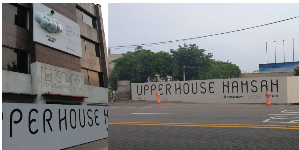
<Figure 6.13> Construction area for new gated housing unit brands, expanding from Seorae Village
