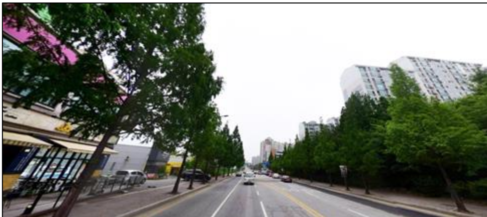
Figure 4.10 Street view of a boulevard in the study area obtained from Naver Corp., Seongnam, South Korea ( http://map.naver.com )
