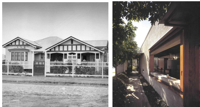
a) Queensland House with a short-ridged roof and a generous wraparound verandah
