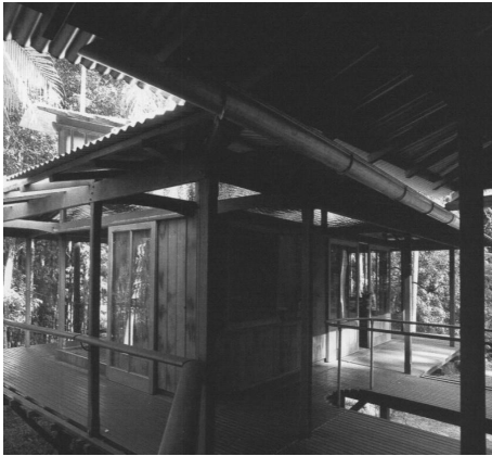
Figure 19. Roofed corridor penetrate through the forest, generous verandah spaces brings light into the house to intergrate architecture with nature
