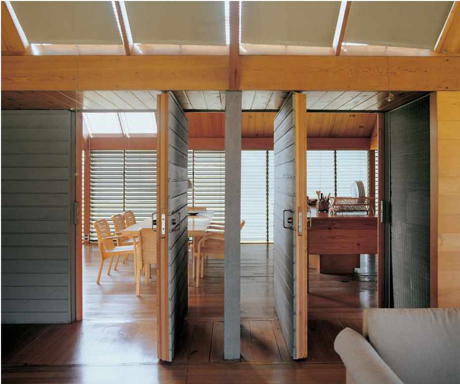
Figure 52. The timber interiors : thick pivot doors
