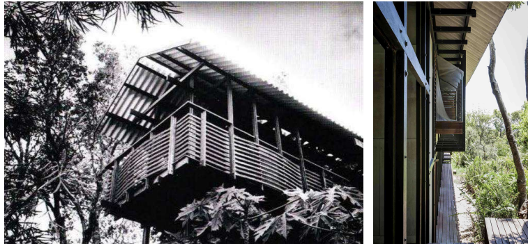
a) Cantilevered verandah space at the upper level b) Attached 'bed box'
