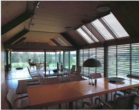
Figure 28. (H2) : Adjustable shading devices Figure 29. (H6) : Retractable Shutter
