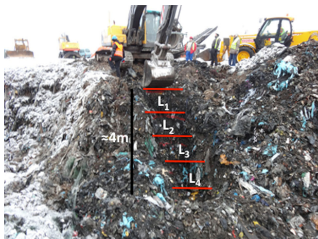
Fig. 1 Excavation of test pit 1 (TP 1 ) with excavation layers indicated with red lines
