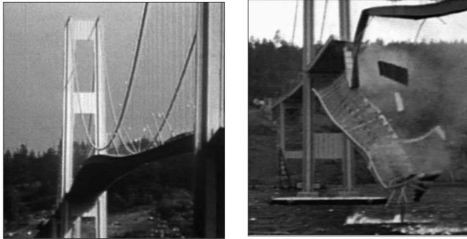
Fig. 1-1 Collapse of Tacoma Narrows Bridge (Fuller et al., 2000).
