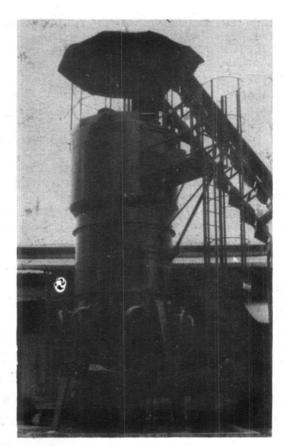
The technology has been primarily applied in the provision of process heat for drying cut coconut kernels for desiccated coconut manufacture. Other applications of the technology for process heat include: (a) sterilisation of coconut kernels; (b) drying parings; (c) drying freshly cut coconut meat - thus by-passing copra production for the manufacture of good quality oil; (d) copra production and (e) firing multi-fuelled
