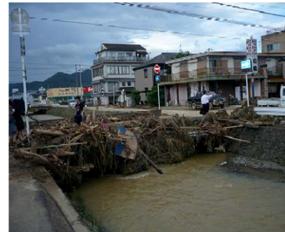
Fig. 1 Log jam formation around the bridge (Sep. 2014, Fukuchiyama city)
