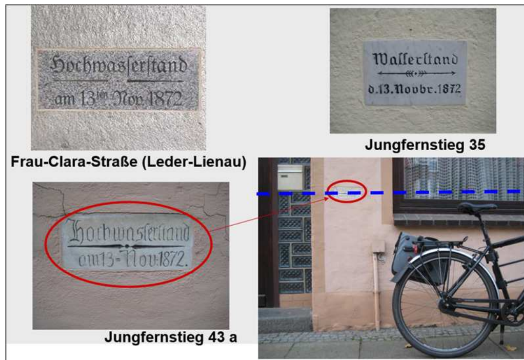
Figure 7: Flood marks in the historical town center of Eckernförde (photos: M. Hamann).
