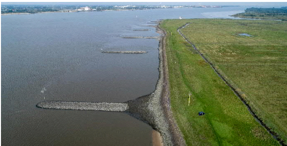
Figure 1 - Prototype recessed groyne in the estuarine waterway of the Lower Elbe, Germany.
