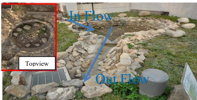
Fig. 3 The experiment site of bio-retention pond next to office building
