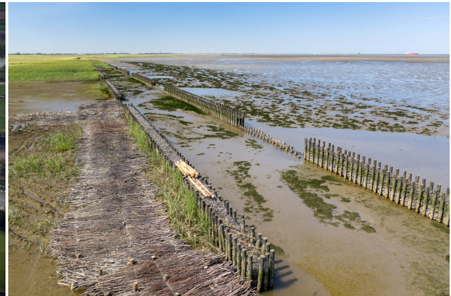
Figure 9: Nature based erosion defences like this gabion-filled wooden stake piling and brushwood mattresses need to withstand ship-induced loading. (Source: German Federal Waterways Engineering and Research Institute).
