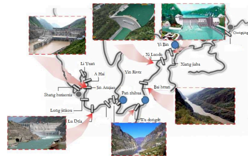
Fig. 9 Dam constructions on the upper Yangtze River
