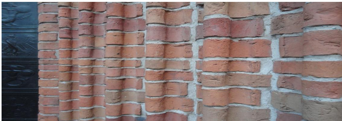
The munkensten brickwork typology.
