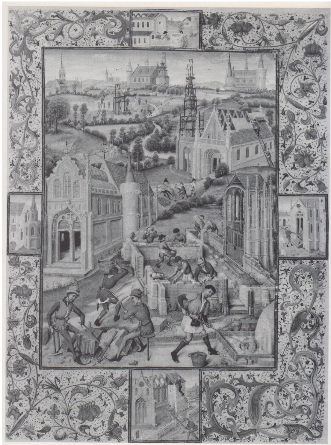
A miniature of 1460 depicting a stonework site (Austrian National Library of Vienna).
