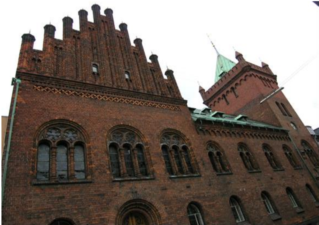
Backstein brickwork in Helsingør's administration building.
