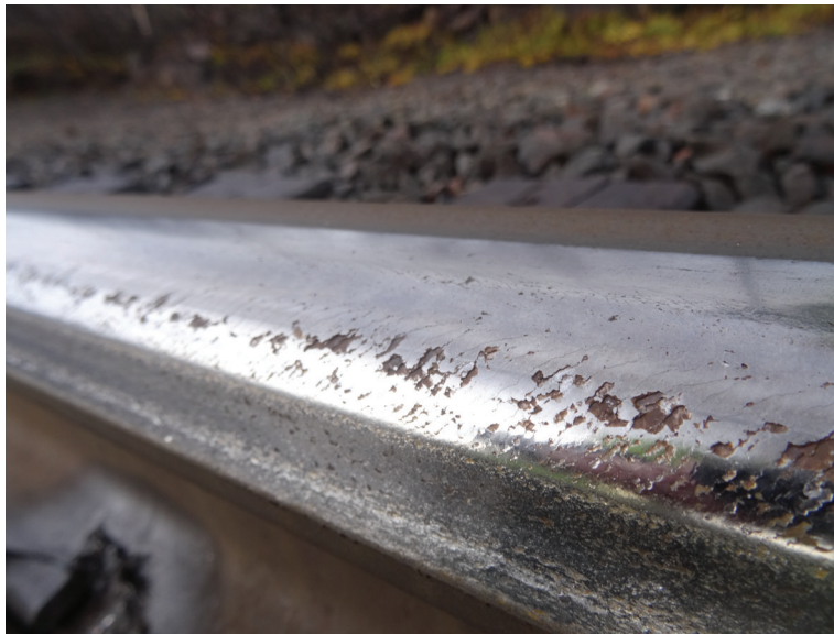
Figure 1.1: Gauge corner RCF cracks of a rail. Photo: Anders Ekberg.
