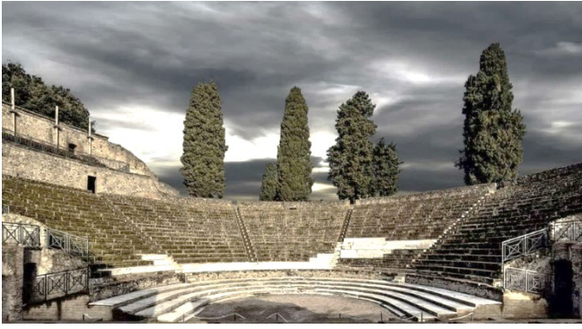
Fig. 8. View of the Roman theatre of Pompeii highlighting the presence of the ambulatory and the gallery on the western side of the cavea .
