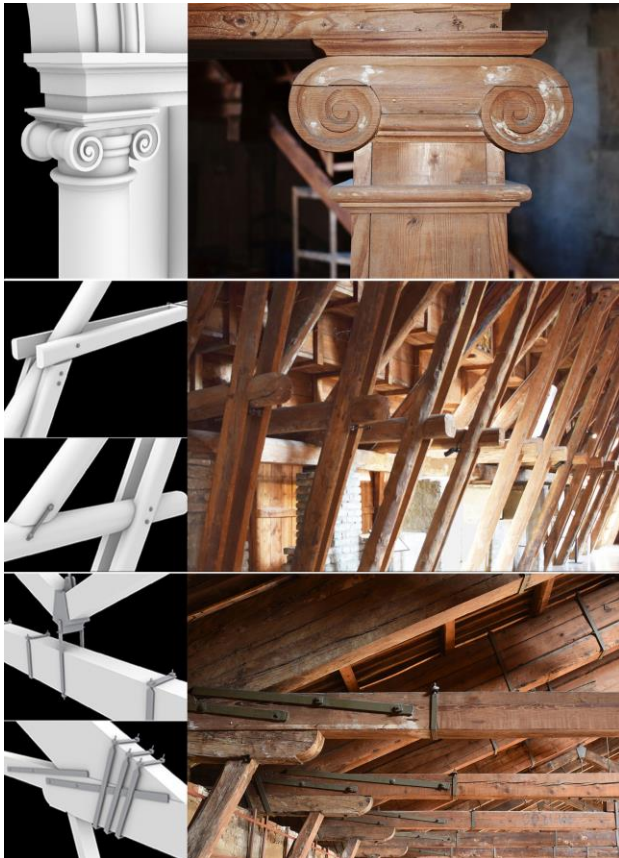
Figure 4. Photographs and digital reconstructions of some classes of elements present in the Farnese Theatre in Parma.
