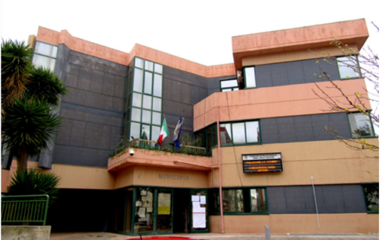
Figure 2. Principal façade of the “Municipal Headquarters” of Palagianello.
