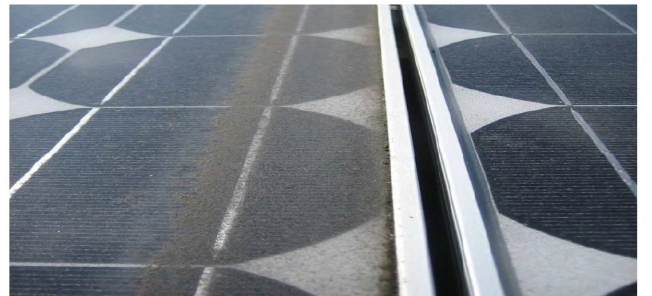
Fig. 7. Dust deposition on the PV panels.
