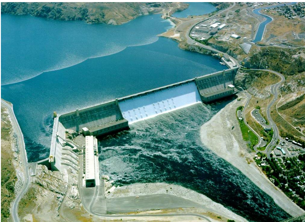
Source: Grand Coulee Dam.jpg
