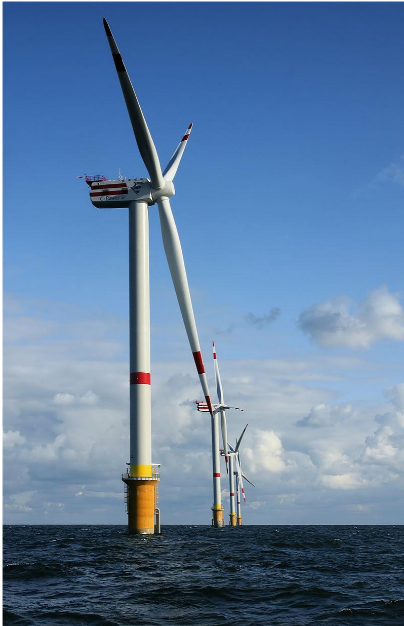
Fig. 6 Offshore wind farm, using 5 MW turbines REpower 5M in the North Sea off the coast of Belgium.
