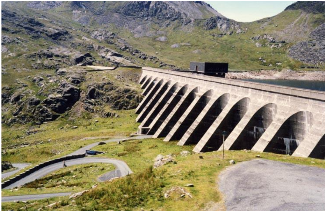
Fig. 15 Pumped-storage hydroelectricity – the upper reservoir (Llyn Stwlan) and dam of the Ffestiniog Pumped Storage Scheme in north Wales. The lower power station has four water turbines which generate 360 MW of electricity within 60 seconds of the need arising
