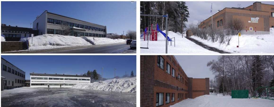
Figure 4.3 School T (left) and School C (right) photographed from the street and the schoolyard.
