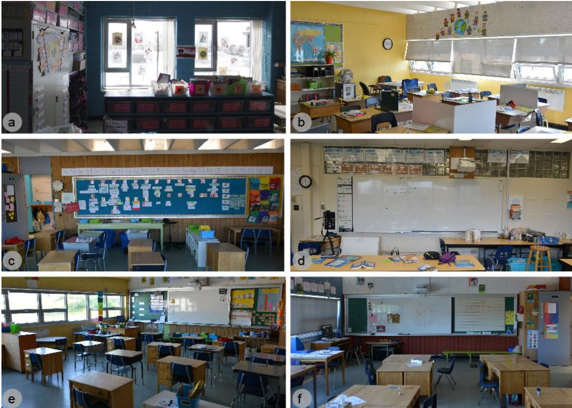
Figure 3.12 Physical traces of occupants' adaptive behaviour revealing their control of natural light, electric lighting, outdoor views and natural ventilation. (a) Storage unit making opening windows more difficult (b) Shades reducing solar gain, yet preventing efficient natural ventilation (c) Teaching material influencing surface reflectance (d) Teaching material on transoms affecting borrowed light in corridor (e) Organisation of students' desks enabling outdoor views (f) Organisation of students' desks with their backs to or facing the window.
