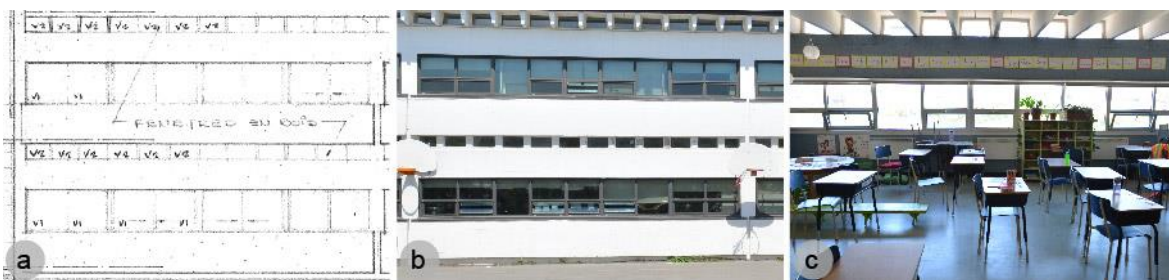
Figure 3.11 Window replacement reducing thermal and auditory exchanges between classrooms and schoolyard. (a) Elevation of the original construction (b) Exterior facade in June 2019 (c) Classroom in June 2019.
