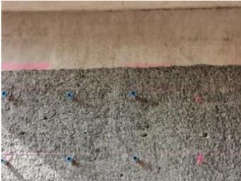
Figure 41. Visual inspection of the pier south face of the study bridge (Stripped degraded surface for repairs)
