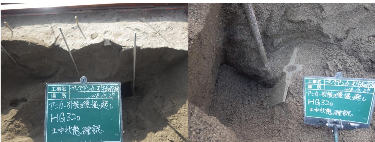
(c) HG320 anchor at w = 250 mm
