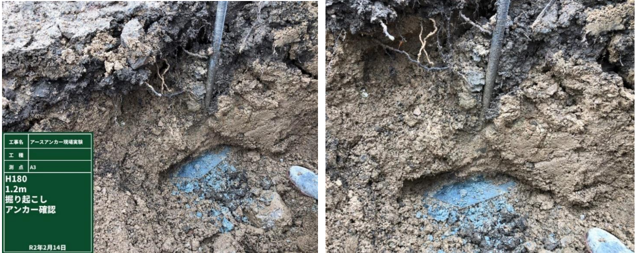
(a) HG180 at A3, H = 1.2 m at w = 650 mm
