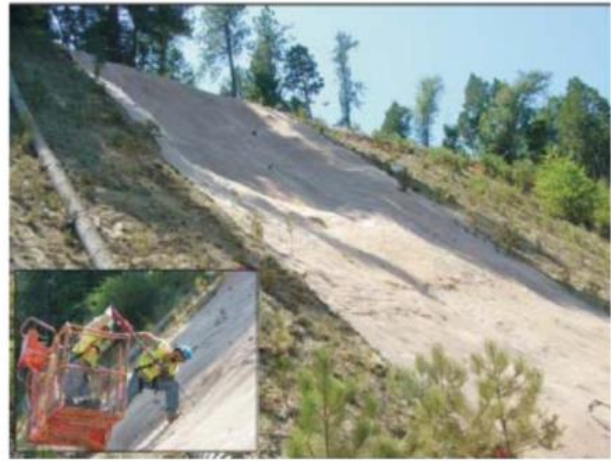
(b) Slope repair using earth anchors
