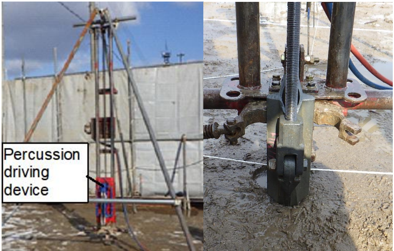
(a) Driving device of flip anchors
