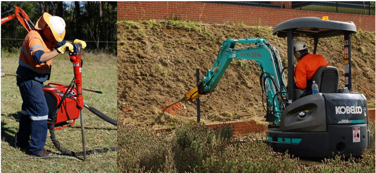
Fig. 1.3. Installation of flip anchors (Anchoring Rope and Rigging Pty Ltd., 2021).
