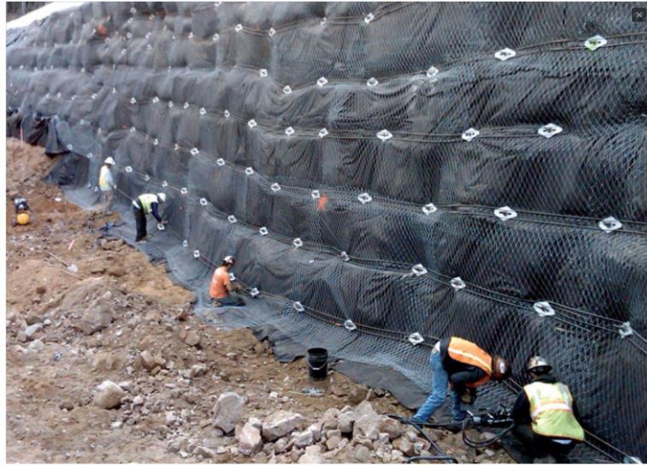
Fig. 2.38. Application of flip anchors (Mantaray anchors) to support a slope along Guanella Pass (Williams Form Engineering Corp., 2021).
