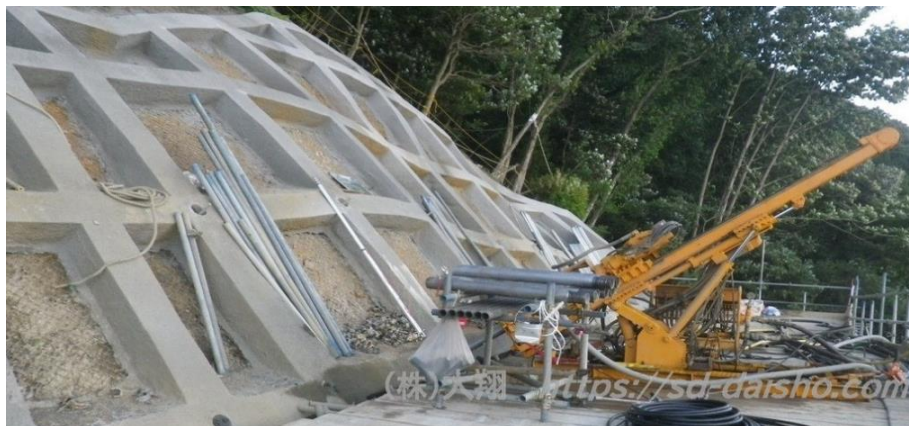
Fig. 1.10. Construction (drilling) of soil nails (Daisho Co., Ltd., 2021).
