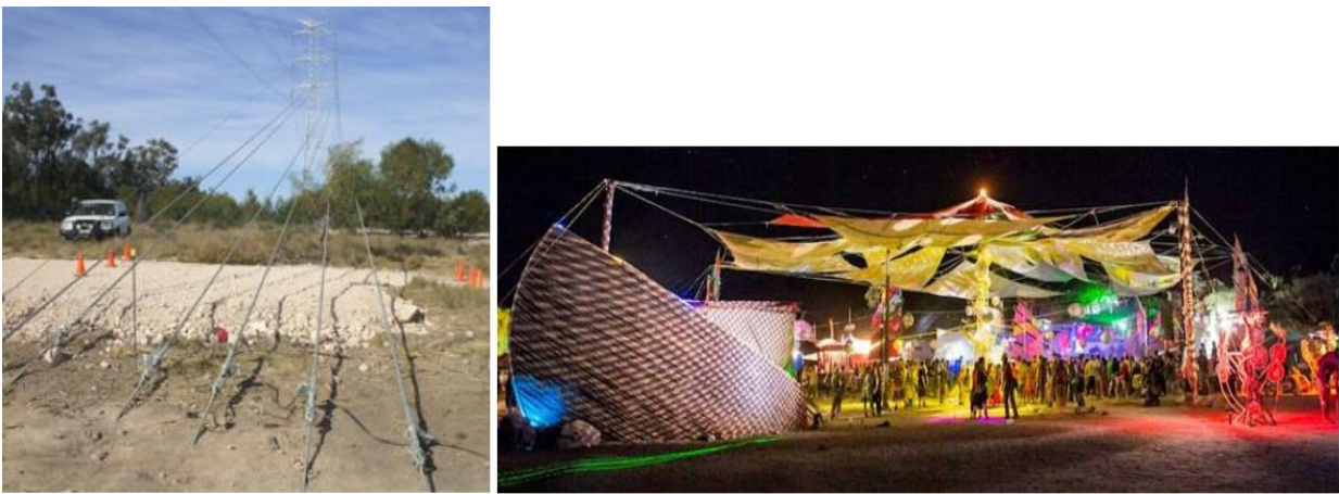
Fig. 2.36. Application of flip anchors (HULK anchors) to support transmission tower, tents for festival (Anchoring Rope and Rigging Pty. Ltd., 2021).
