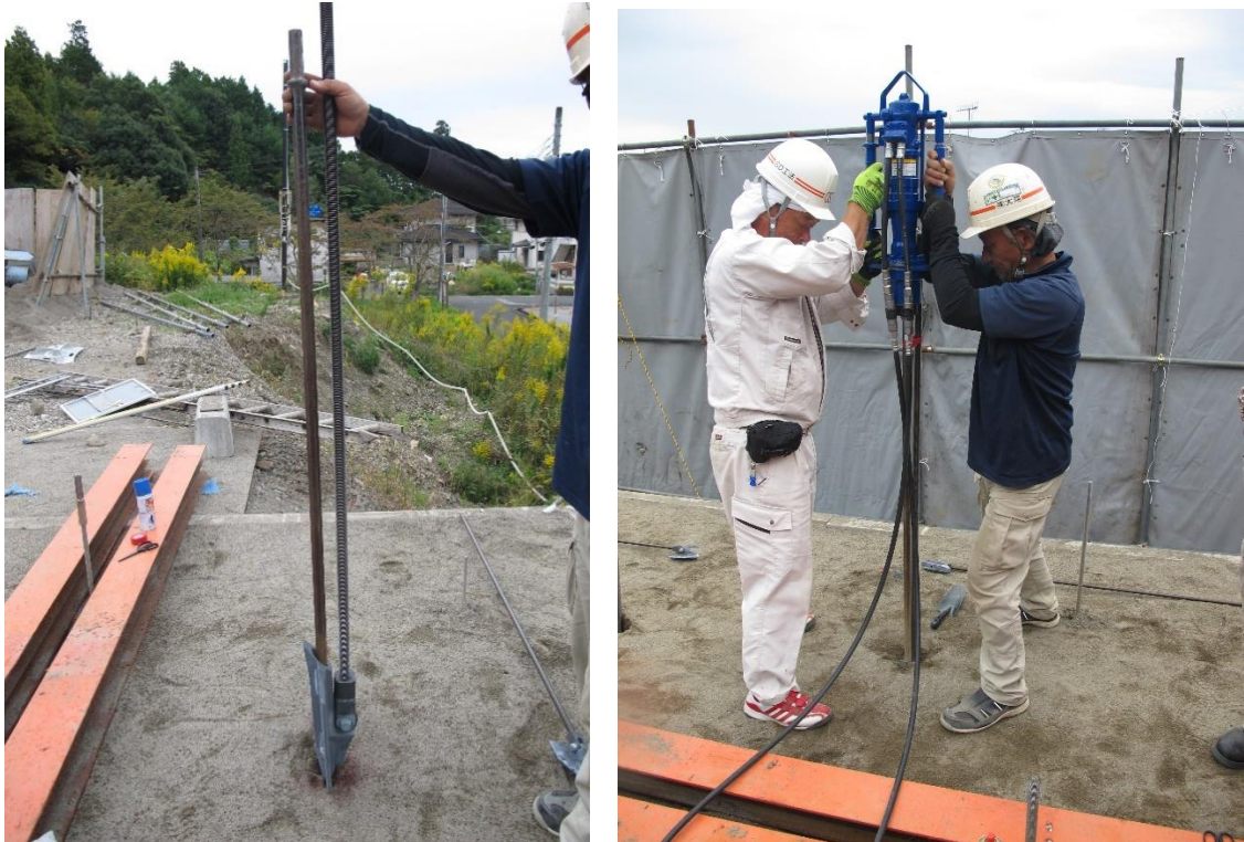
(b) Installation condition of Driven anchors
