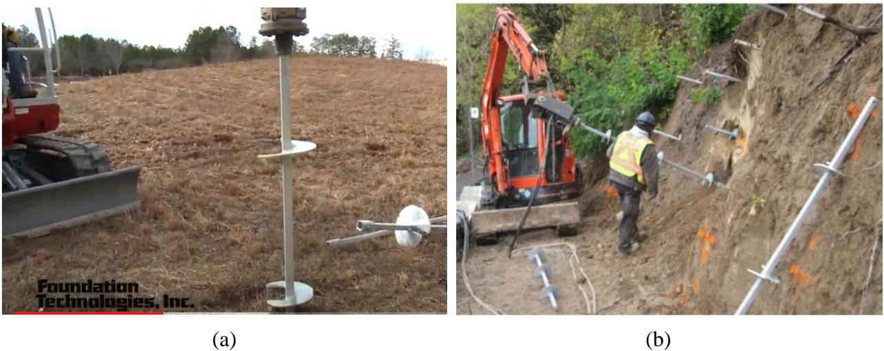
Fig. 1.4. Helical anchors (piles) by (a) Foundation Technologies Inc. (2021), (b) Lazarte et al. (2015).
