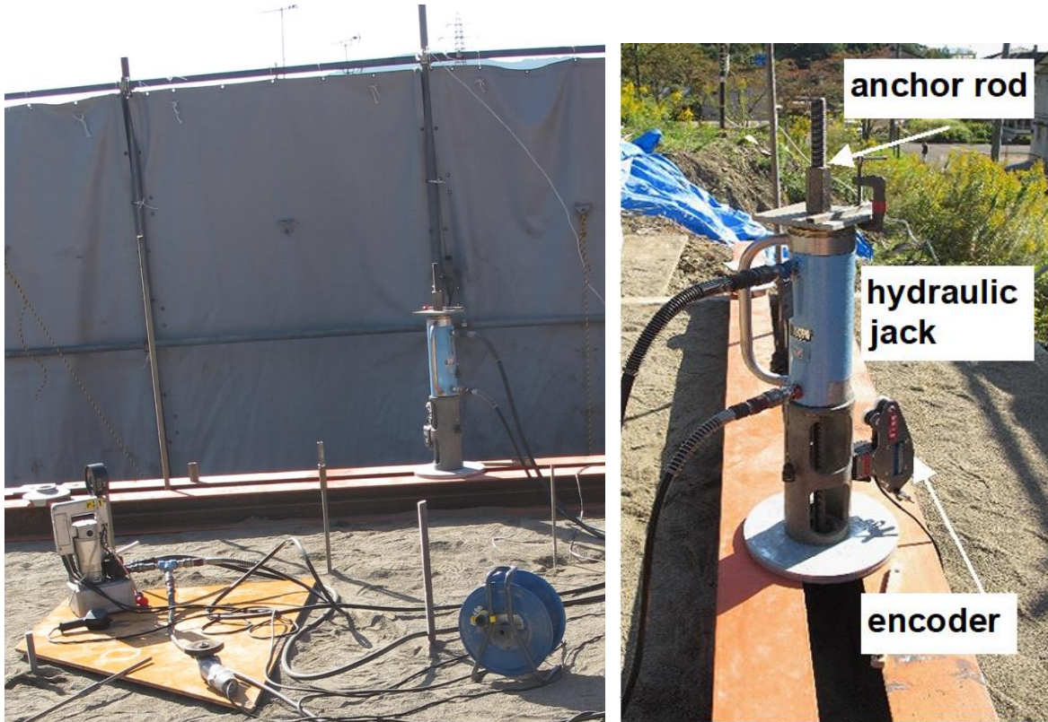
Fig. 3.36. A set-up for pulling-out anchors.
