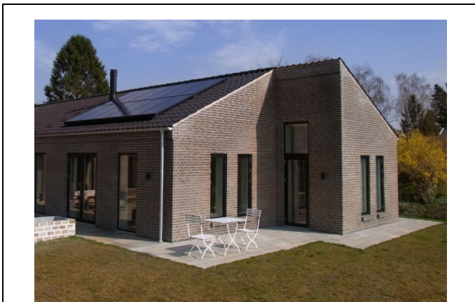
Figure 4-47 A typical new Danish low-energy house. The house is more complicated to operate than an older house due to the larger number of technical installation.
