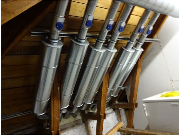
Figure 3-7 Supply air ducts in attic with flow regulation dampers, silencers and penetration to the outside of the exterior wall.
