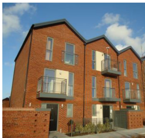
Figure 4-56 Outside view of the monitored dwellings.
