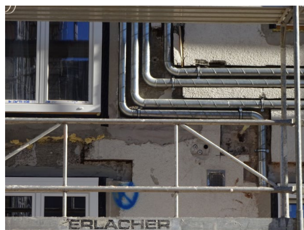
Figure 3-3 View of supply air ducts being routed on exterior wall prior to installing new insulation layer.
