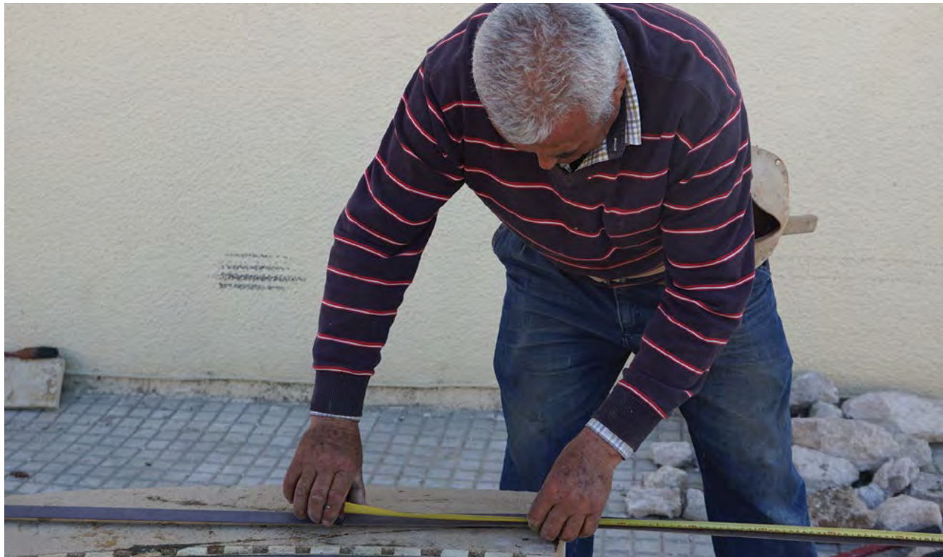
Local concrete foreman preparing the formwork of the main bench
