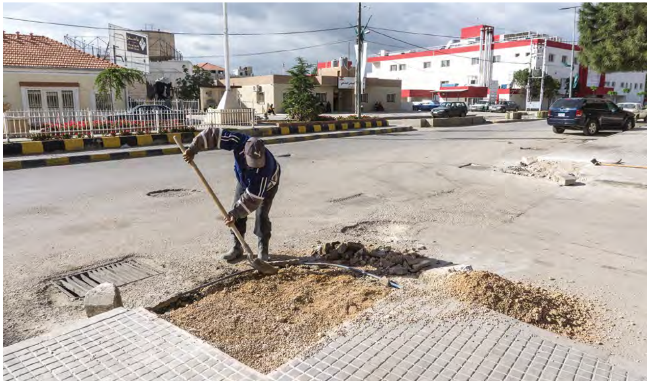
Local concrete worker preparing to pour the access ramp
