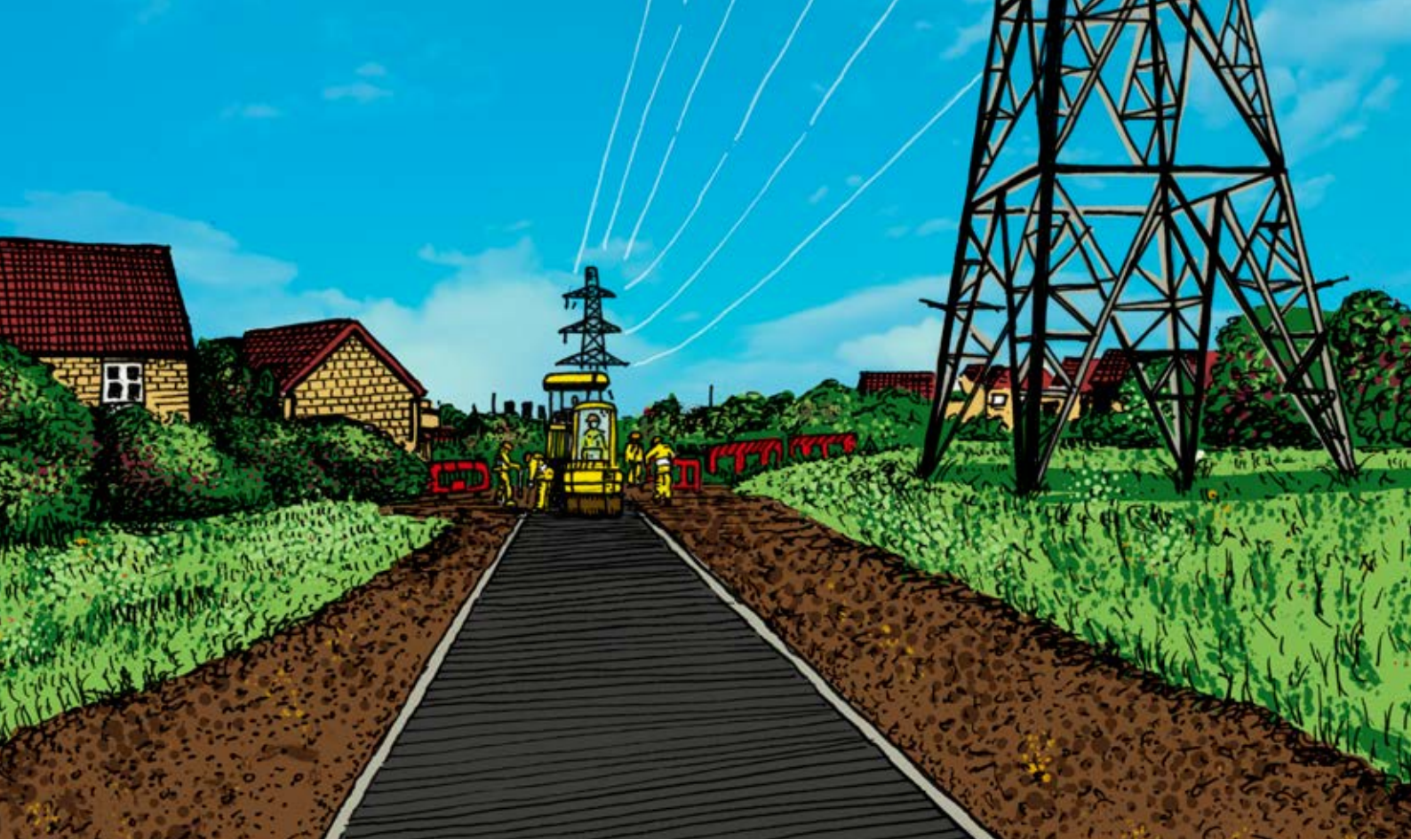
A bike path under construction in a new development. © WITPI
