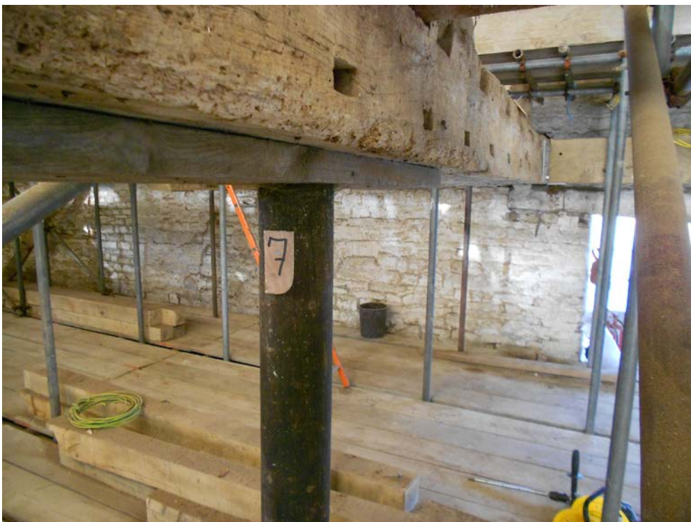
Figure 5: Floor beam 7, sampled as wrh06 and wlf03, photo Martin Bridge
