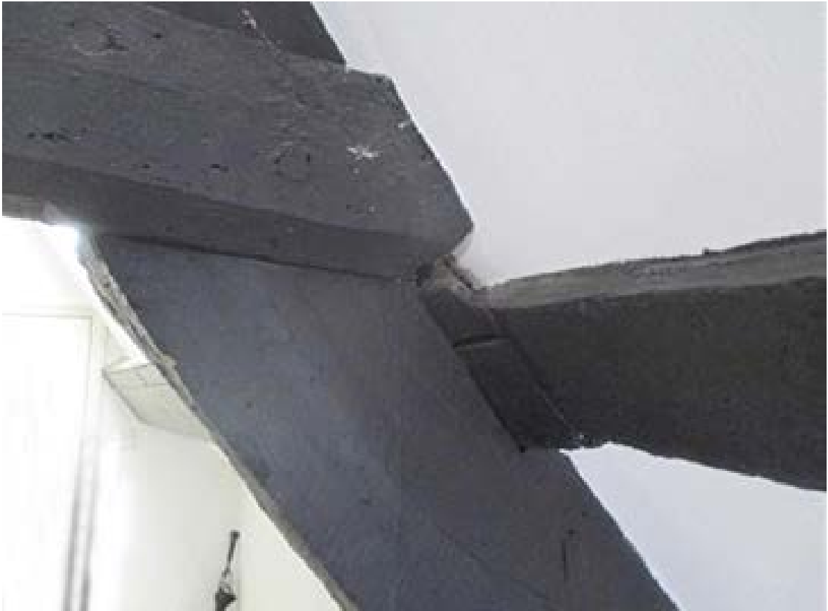
Figure 3: Detail of truss, showing the collar pegged over the principal rafter, and the lower purlins crudely scarfed over the principal rafter and slightly trenched (photograph Martin Bridge)
