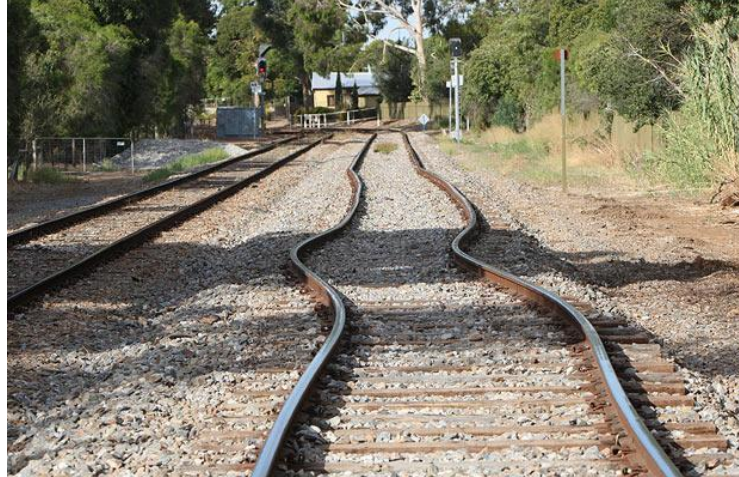
Figure 3.8 Asymmetrical buckling shape (Clark, 2018).
