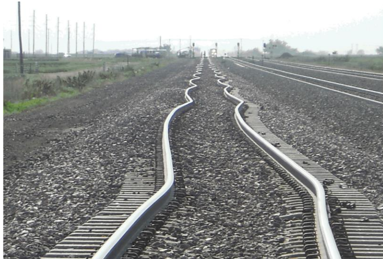
Figure 3.8 Asymmetrical buckling shape (Clark, 2018).
