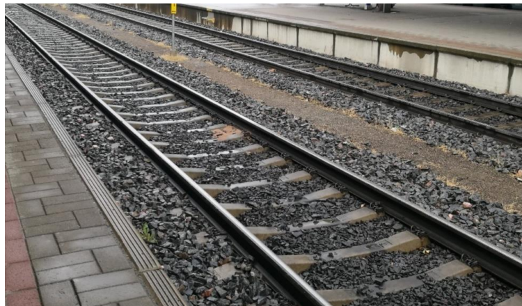
Figure 2.3 Ballasted railway track with concrete sleepers.
