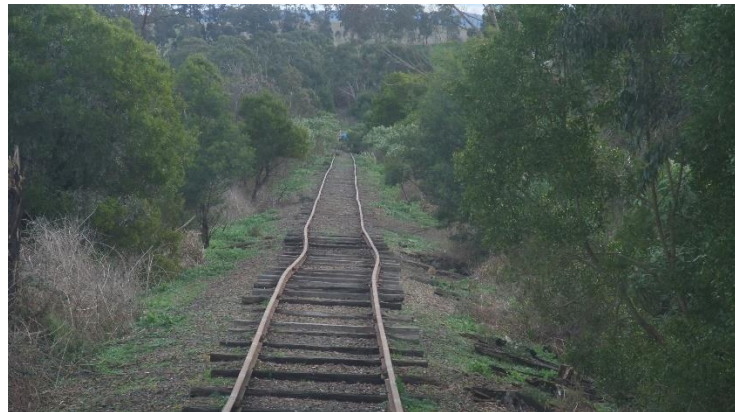
Figure 3.7 Symmetrical buckling shape (Lankyridner, 2014).
